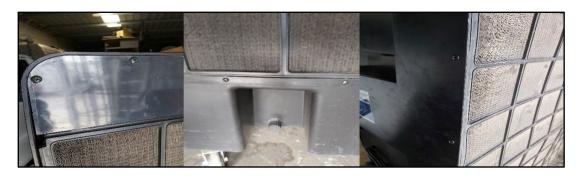
4. Use a water supply hose to manually fill the reservoir to the full level on the level indicator panel located at the rear of the unit below the air inlet panels, or if overfilled drain off the excess water to the correct full level.
